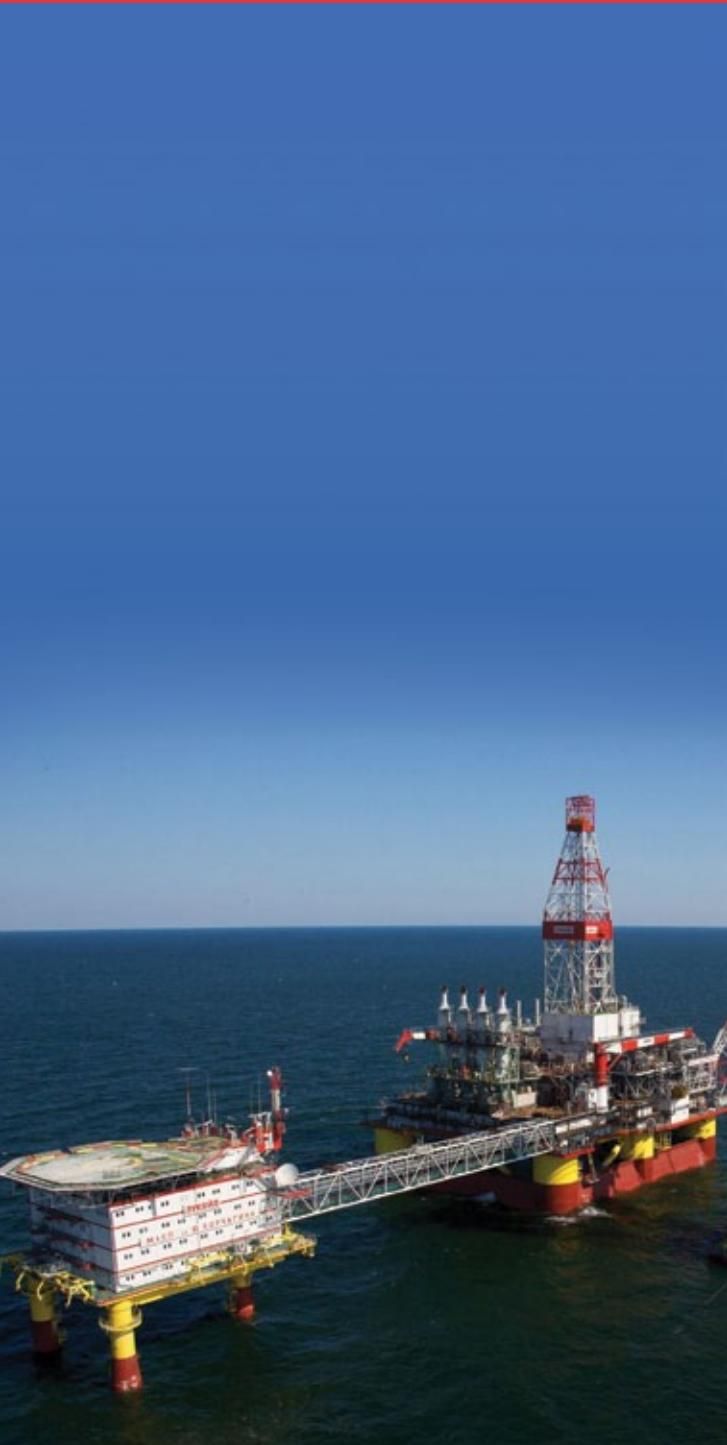
The OTF includes a floater and a single point mooring (SPM). The facility is designed to load 10-12 ths tn deadweight shuttle tankers with crude to ensure the delivery of crude from the Yury Korchagin field.
