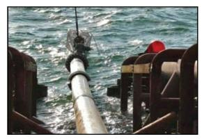
The oil is fed from the LSP-1 to the marine transportation complex using 58 km of nonembedded pipeline, 300 millimeters in diameter with walls 16 mm thick.
