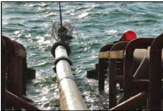
The oil is fed from the LSP-1 to the marine transportation complex using 58 km of non-embedded pipeline, 300 millimeters in diameter with walls 16 mm thick.
